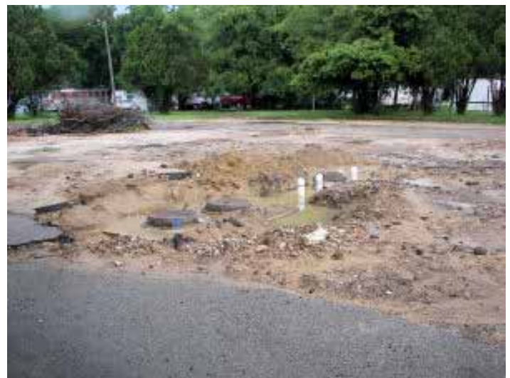
New Plumbing work?
