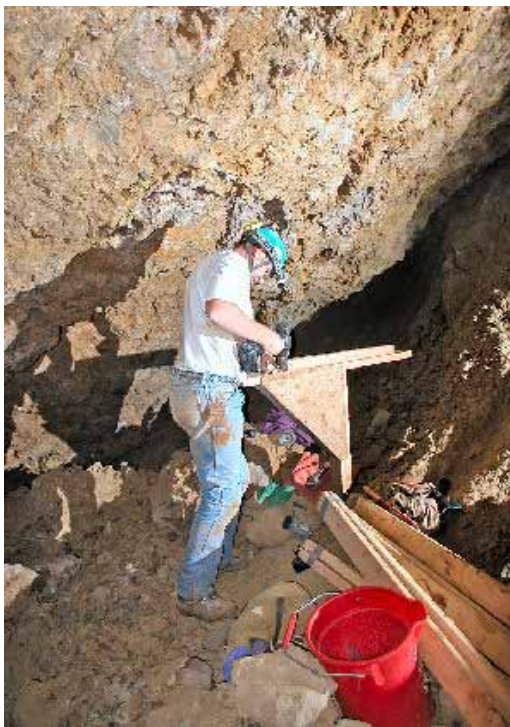
Steve Peerman assembles the next section of the wooden casing for the shaft.
