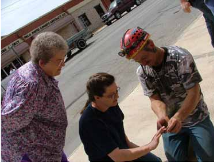
Wayne Peplinski shows the building owners bats that he's removed from the building.
